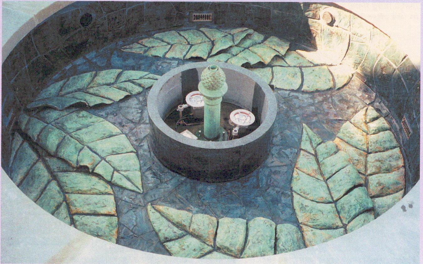
Water will shoot up from the central pedestal, fill the granite cylinder, drizzle over the edge, and cover the leaves with 3" of water.
